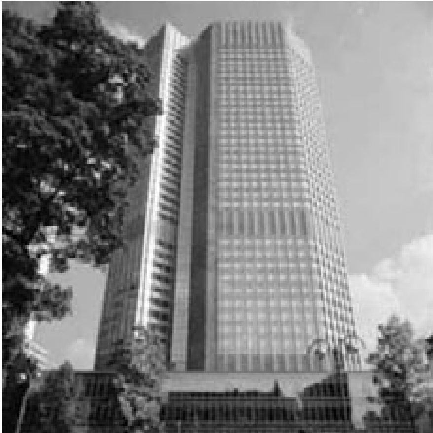
Eurotower Building, sede del Banco Central Europeo, Frankfurt-AmMain, Alemania.
